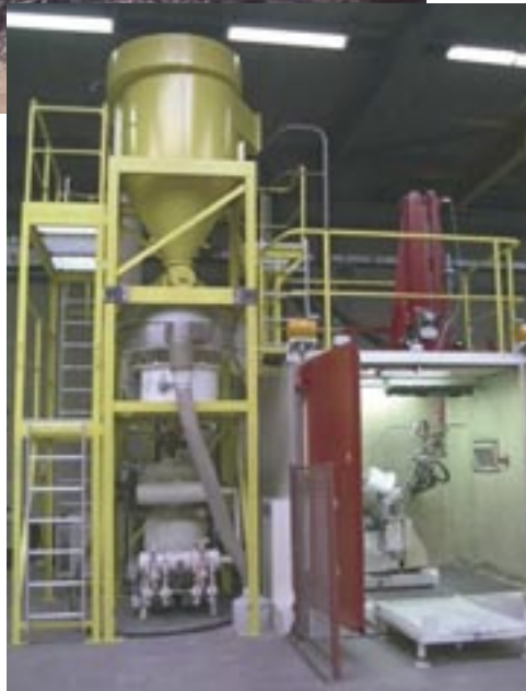
Cyclone application for the recycling of glass beads in a shotpeening process for airplane wheel-rims. Capacity: 3,600 m 3 /h.
