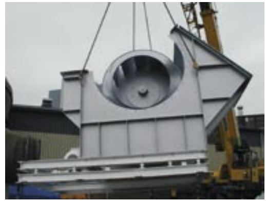
Assembly of a flue gas fan type A 80 3 / 4 . Capacity: 250,000 m 3 /h.
