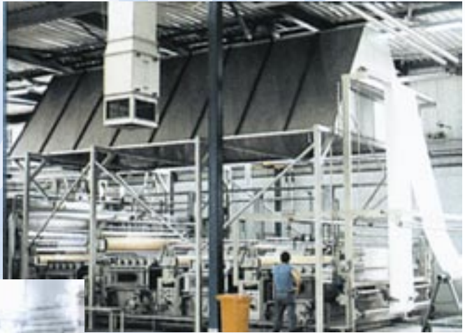
Exhaust installation for vapour extraction in textile industry Suction-hood fabric stainless steel AISI-316: 22 x 4 meter Exhausted capacity: 72,500 m 3 /h
