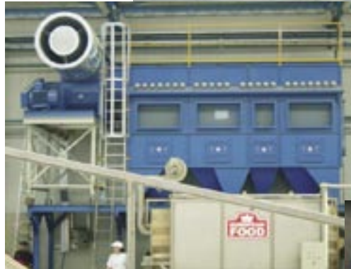
Cartridge filter type 48/21 with cloth surface of 1,008 m 2 . Application: exhaust of a production line Snack-factory. Capacity: 60,000 m 3 /h
